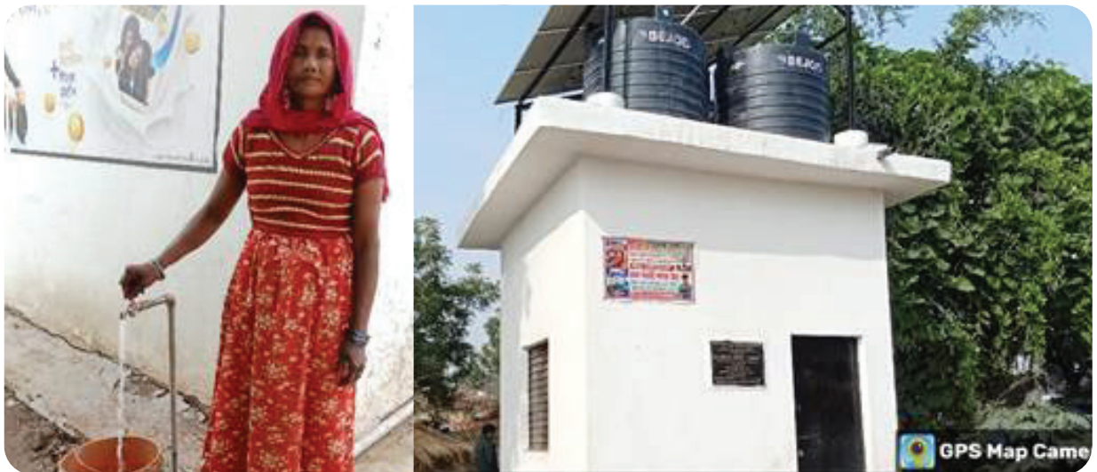
Submersible Pump - Majhawan
