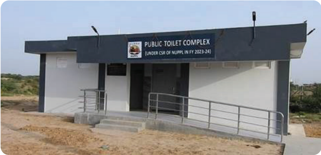
NUPPL constructed Public Toilet at NUPPL Arch Gate
