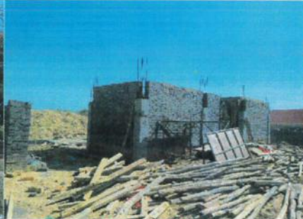
Toilet block beside NH 34
