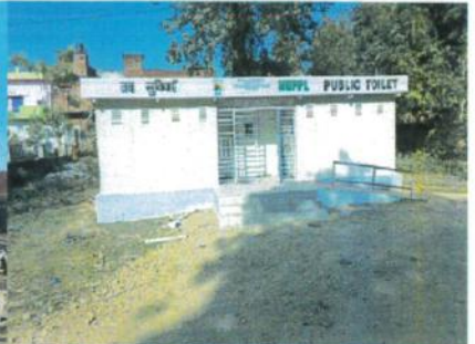
Prefab toilet block at various railway station of Northern railway
